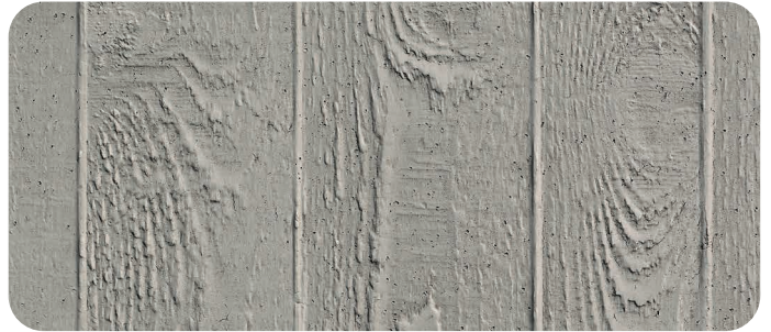
122E Brettschalung | timber formwork
